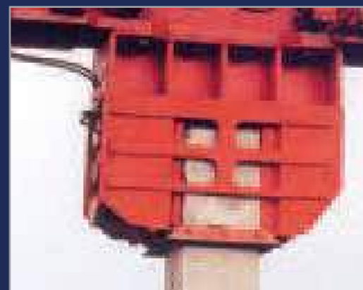
23HFV Vibrodriver extracting 400 mm square concrete piles.
